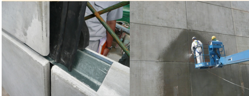
Picture above is our sealant-less solution: TP-600 Compriband Tapes, ME220VV EPDM Membrane with Self-adhesive, and/or ME480 Butyl Tape (for Fire retardant requirements)
